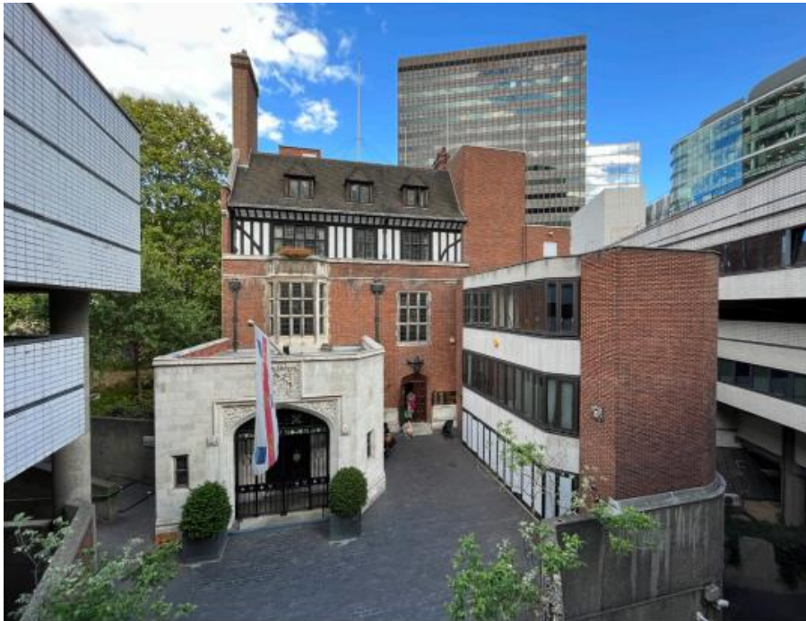
Site photograph Ironmongers Hall existing from existing Highwalk looking east with Bastion House and MoL
